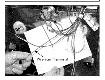
11. Use the wire nut connector provided to connect the power wire that was attached to the 170° thermostat to the #1 wire from the
